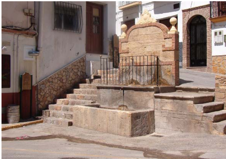
Pilar Barandilla ( http://wikanda.almeriapedia.es )
