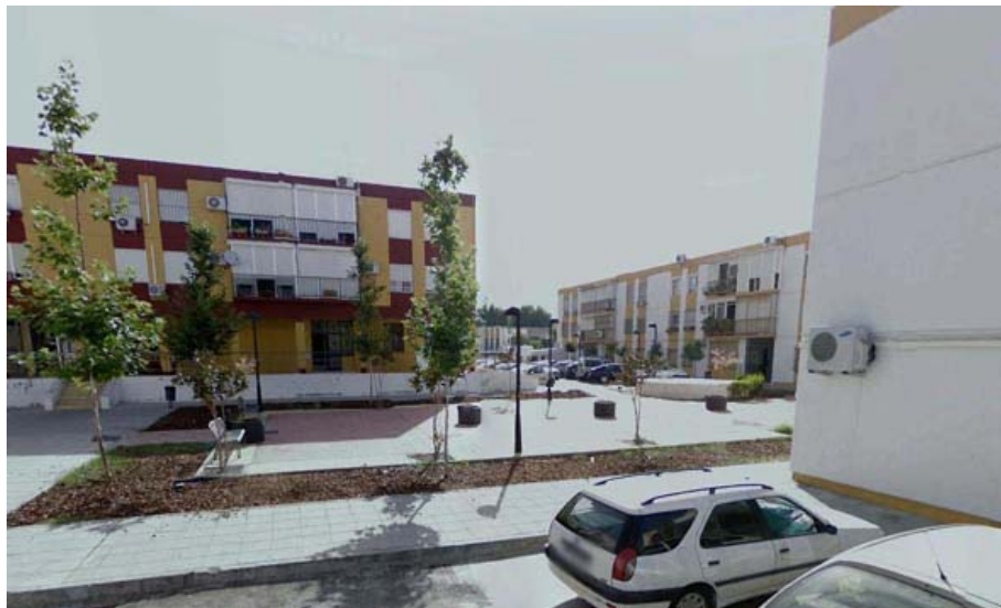
El Pozo (Google Earth-Street View, julio 2008)
